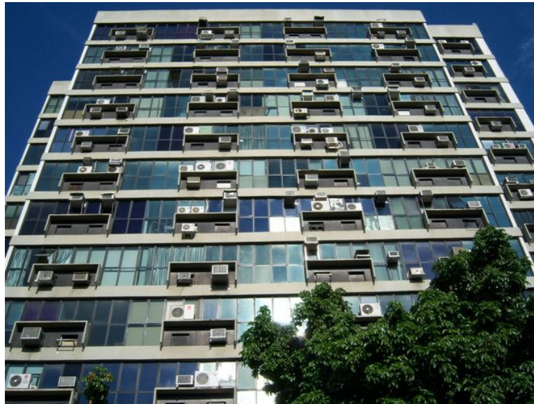
Figure 1.3 - Applied electrically driven compression air-conditioning at a commercial building in Rio de Janeiro - Brazil.
