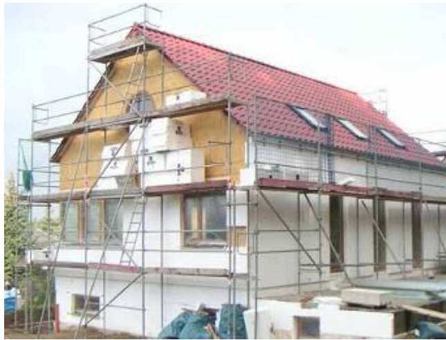
Figure 3.10 - Insulation with EPS Polystyrene plates in Germany. Source: www.netz-gemeinschaft.de/deetz/Tagebuch/Pict5379.jpg
