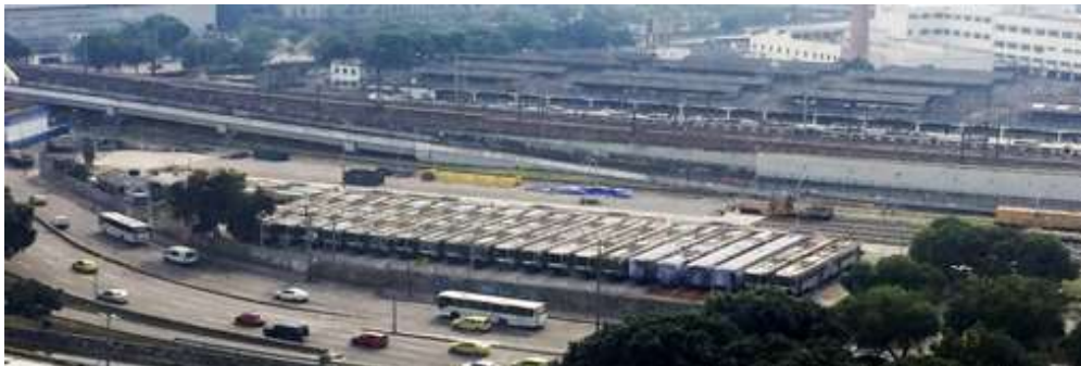
Figure 2: Pre-metro parking, in Metro Rio Garage - Picture taken in 2017 Font: from the Rio de Janeiro Administration building, by the author
